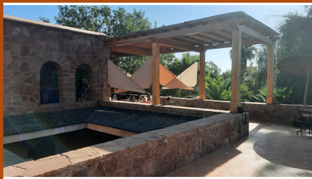
Roof top terrace dining
